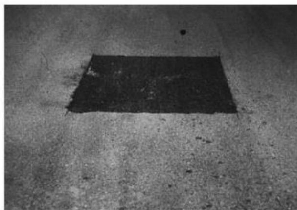
Gambar 2. 23 Tambalan ( Patching and Utility Cut Patching )
