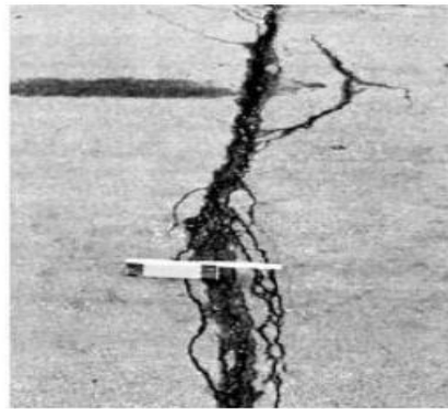
Gambar 2. 17 Retak Sambung ( Joint Reflec Cracking )
