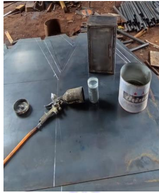
Pengecatan box panel
