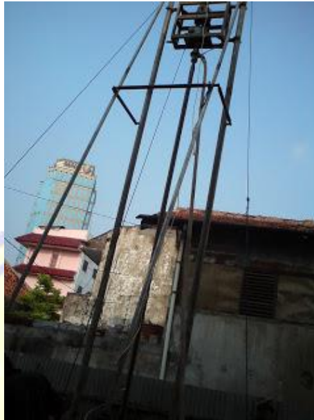
Gambar 2.10 Bored Pile Mesin Gawang
