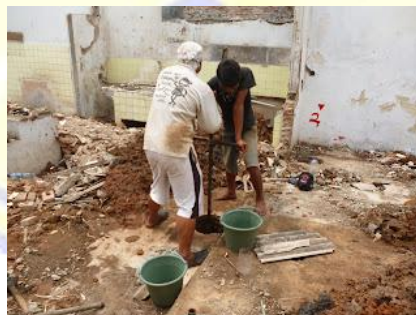
Gambar 2.11 Bored Pile Manual
