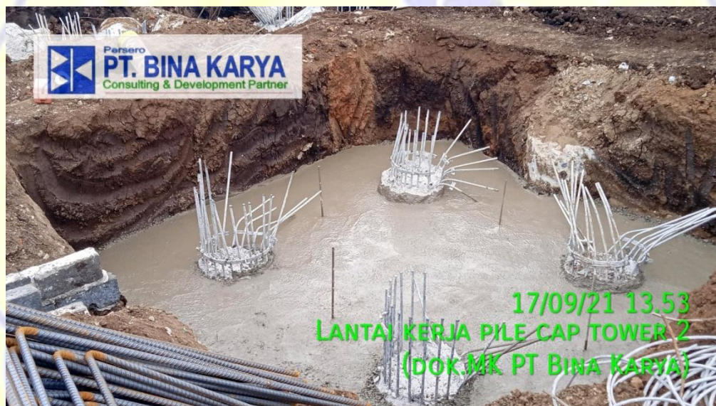
Gambar 2.7 Pondasi Tiang Bor ( Bored Pile )
