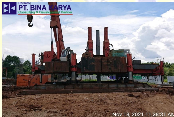
Gambar 2.13 Alat Pancang Hydraulic Static Pile Driver (HSPD)
