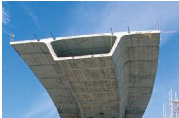
Gambar 2.3 box girder (Sumber: https://pu.go.id/berita/steel-box-girder , 2007)
