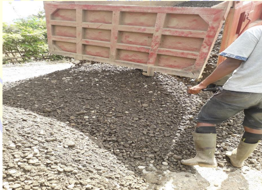
Gambar 2.2. Drop Material LPA
