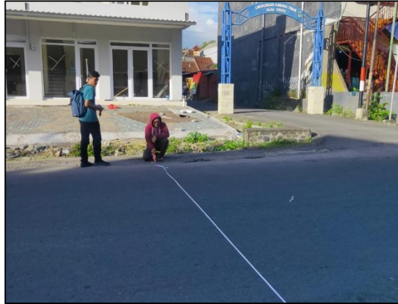
Gambar Pengukuran Lebar Jalan Sta 1+875 – 1+900
