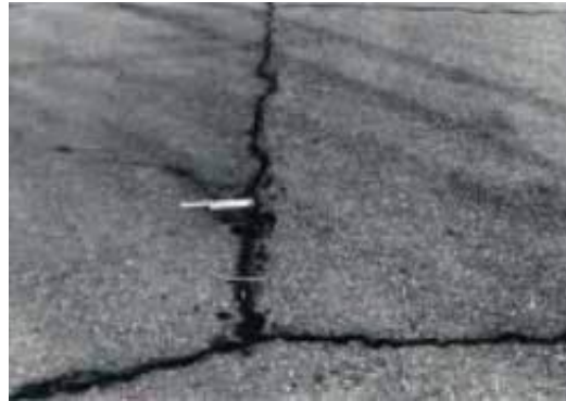
Gambar 2. 15 Joint Reflection Cracking (Retak Sambung)
