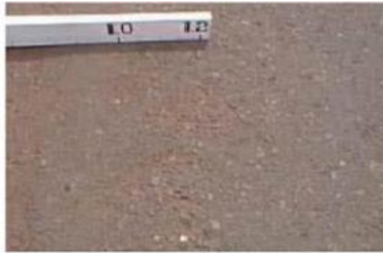
Gambar 2. 23 Polished Aggregate (Pengausan Agregat)
