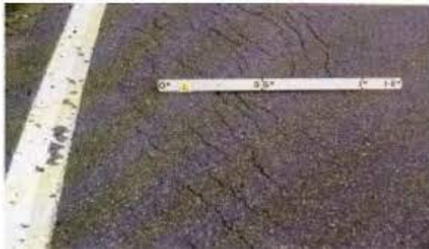
Gambar 2. 33 Slippage Cracking (Retak Bulan Sabit/Retak Slip)
