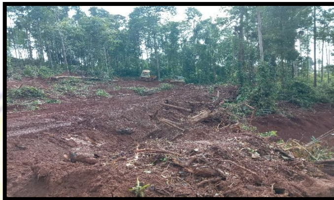
Gambar 2. 2 Proses Land Clearing
