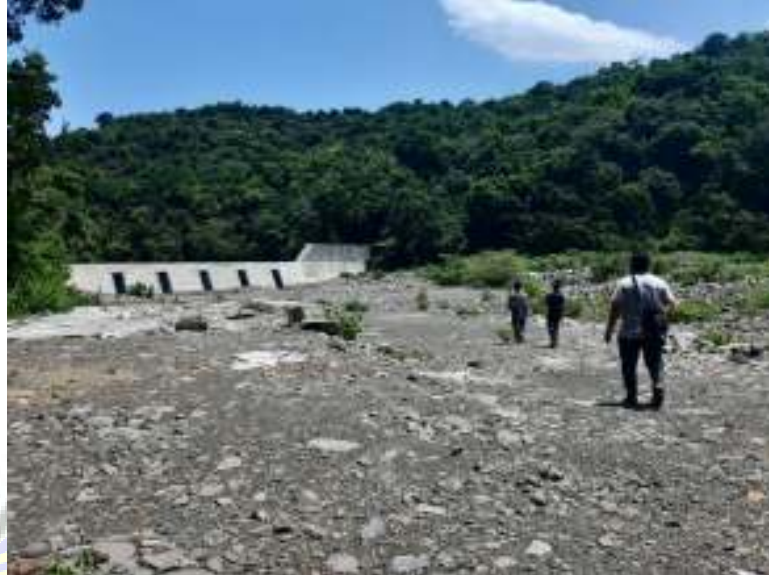
Hulu Sabo Dam
