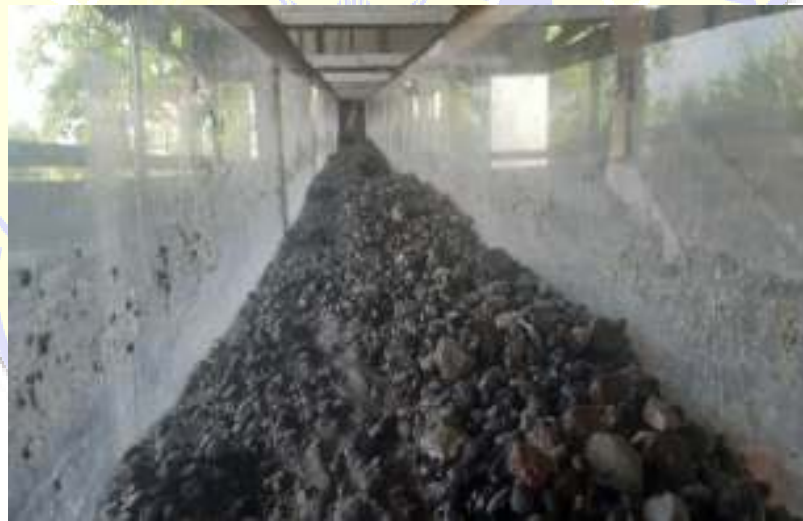
Hulu Sabo Dam
