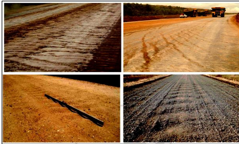
Gambar 2.15 Contoh Kerusakan Jalan Bergelombang ( Corrugated ) (Sumber : Report PT.PAMA, 2015)
