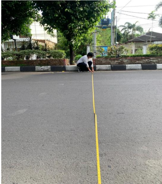
(Gambar D.1: Mengukur lebar jalan)
