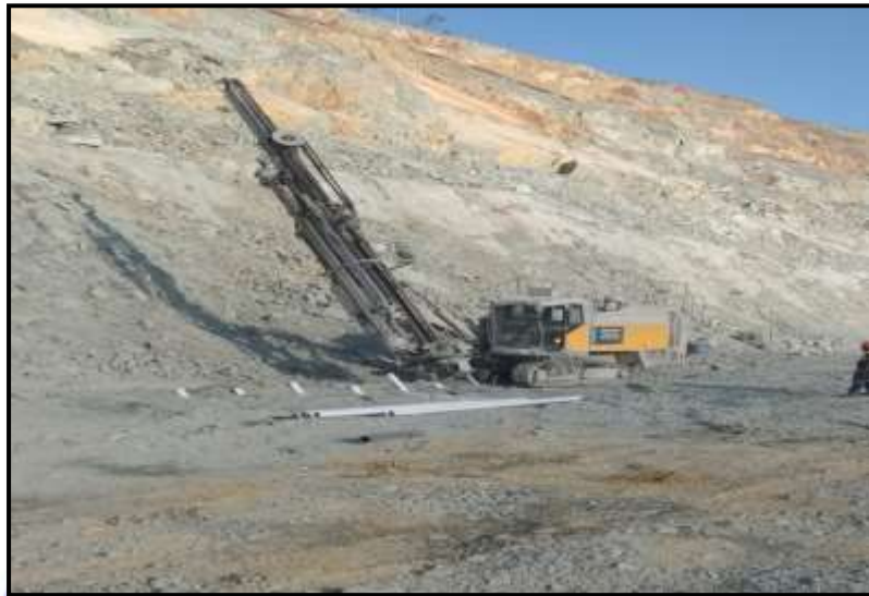
Gambar 8. Small Drill Atlas-Copco D65
