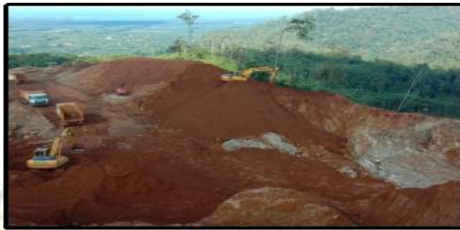
Gambar 2.4 Kegiatan Pengupasan Lapisan Penutup ( Overburden Removal )
