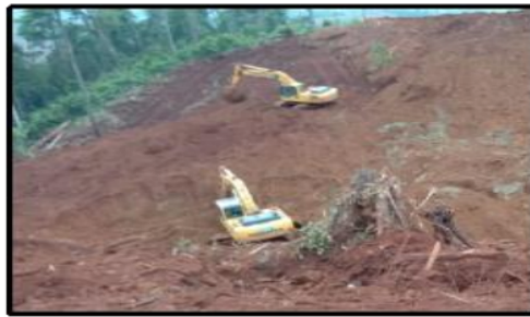
Gambar 2.3 Kegiatan Pengupasan Tanah penutup ( Top Soil Removal )
